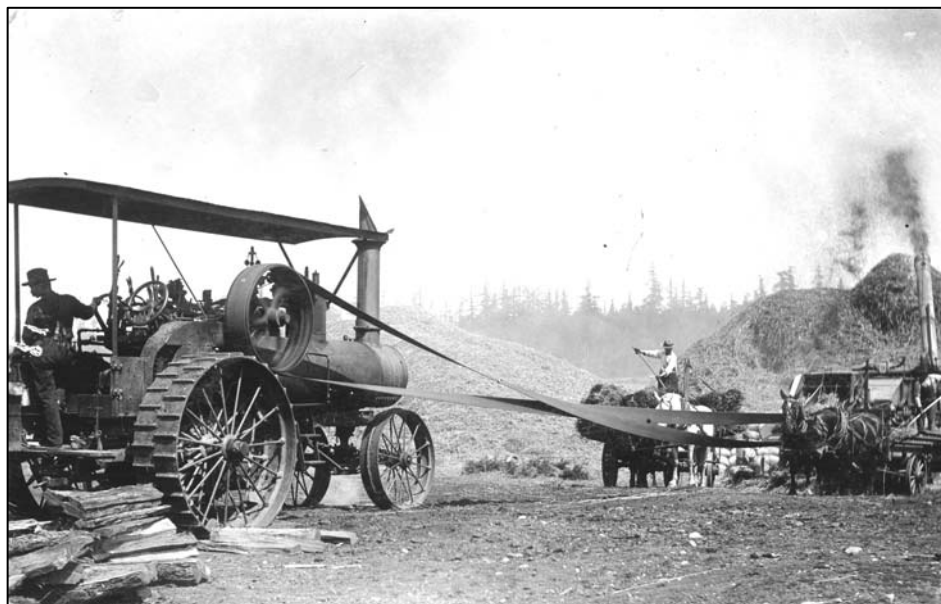
Illustration 8. Threshing on central Whidbey Island farm c. 1900. Note the distance between the steam engine and the threshing machine; the two are joined by a long leather belt. The steam engine was kept some distance from the actual threshing to minimize fire danger. Photograph courtesy of the Island County Historical Society.
