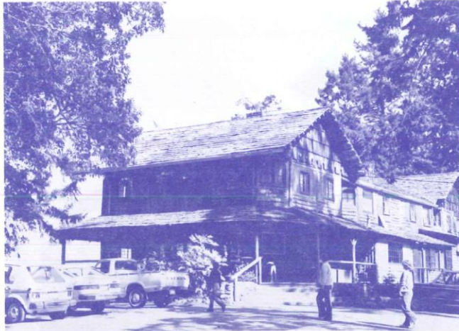
The Captain Whidbey Inn on the shores of Penn Cove (ca. 1901) was constructed from native madrona logs. The Stone family, originally from Nantucket Island, Massachusetts, have made this one of the most popular inns in the northwest.
